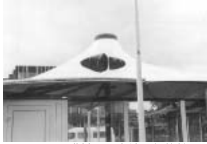
图4 PVC膜材遇明火被局部烧熔
